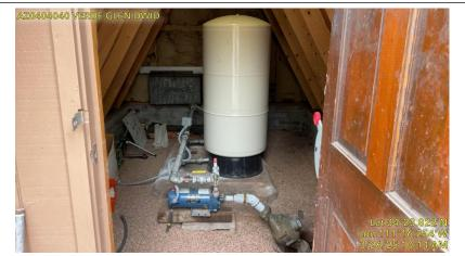
**Photo Description:** 2x bladder tanks and booster station in pump house after EPDS
